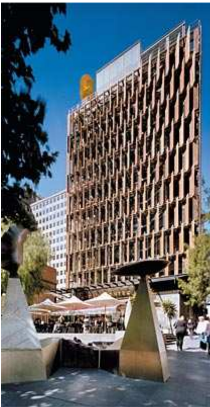
CH2 with shutters open. These automatically open and close in response to sun angle and time of day.
